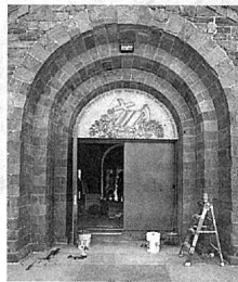
The restored entrance to the Chapel of the Sisters.
